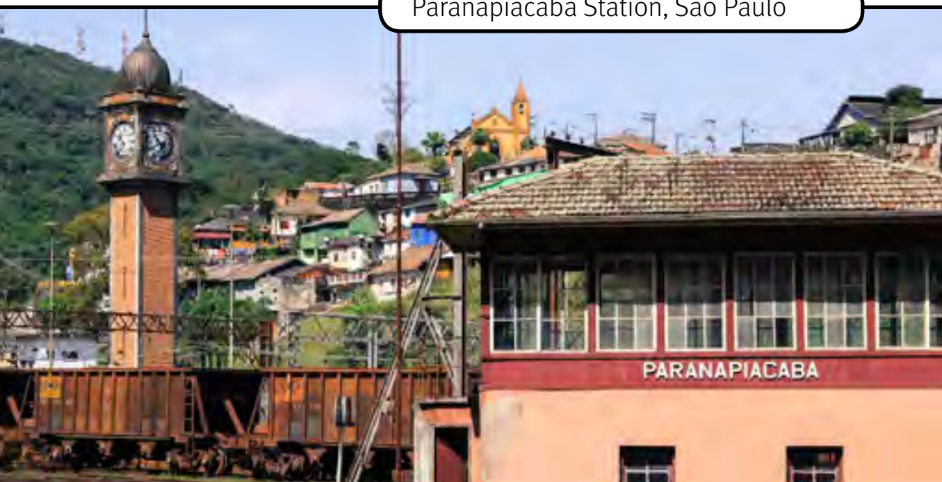
Paranapiacaba Station, São Paulo
